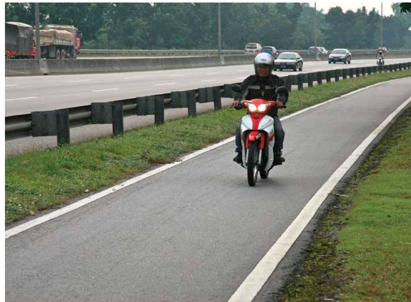
This separated motorcycle lane in Malaysia is a good example of 'forgiving' infrastructure
